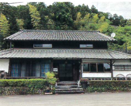
OKUISE WORK (大台町)
